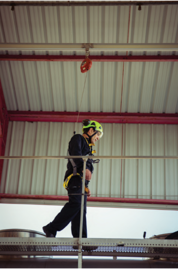
📍 GTLE Lyon, France
